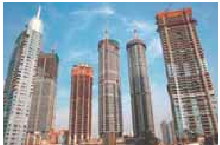
HVAC services for Omkar Realtors & Developers, Mumbai
