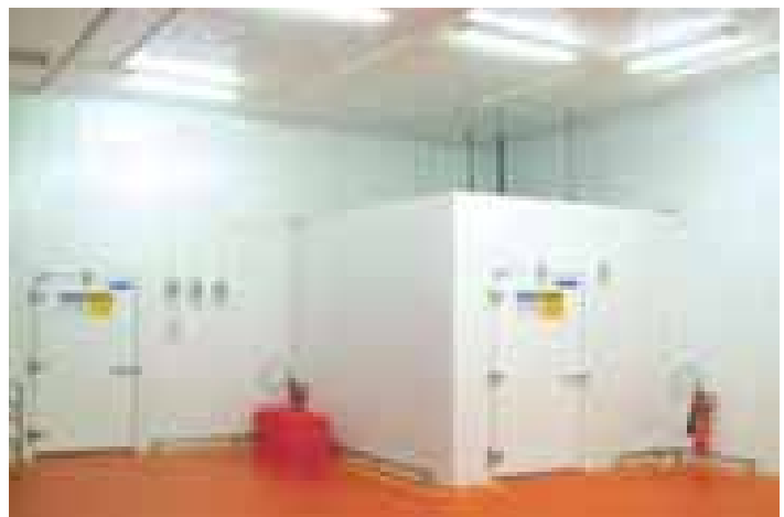
Cold Room installation for Domino's, Kolkata
