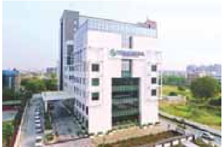
Integrated MEP (Mechanical, Electrical & Plumbing) services for Venkateshwar Hospital, New Delhi
